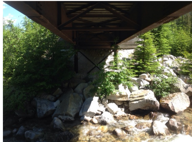
Right Bank Abutment when facing downstream
