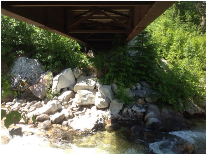
Left Bank Abutment when facing downstream
